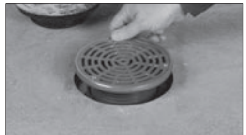
Install Finish Fixture
