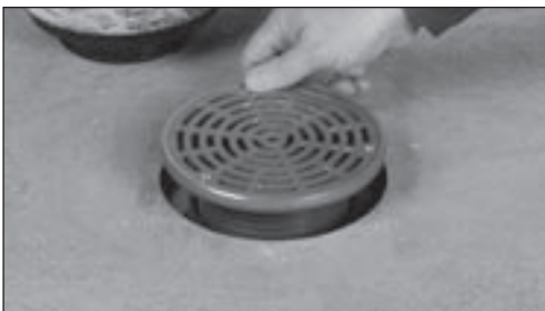
Install Finish Fixture
