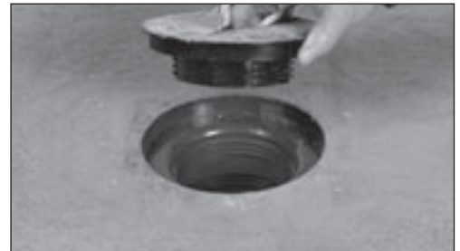
Remove Coring Plug
