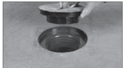
Remove Coring Plug
