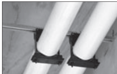
Large pipe: use TouchDown II clamps for pipe up to 2".
