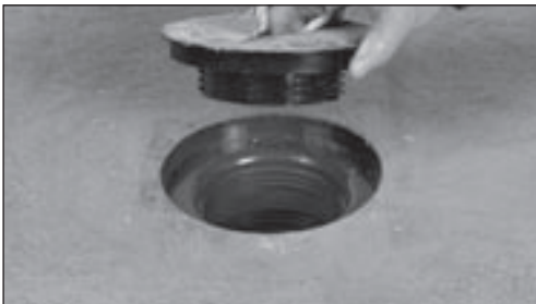
Remove Coring Plug
