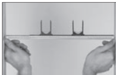
Bend tabs and expand bracket to fit stud bay opening.
