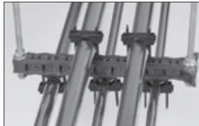
Use 3/8" (#3) threaded rod for trapeze installations.
