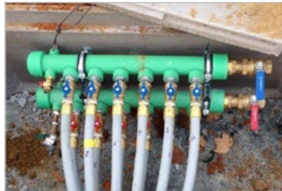
M-8400 GeoGreen™ mounted ground vault.
